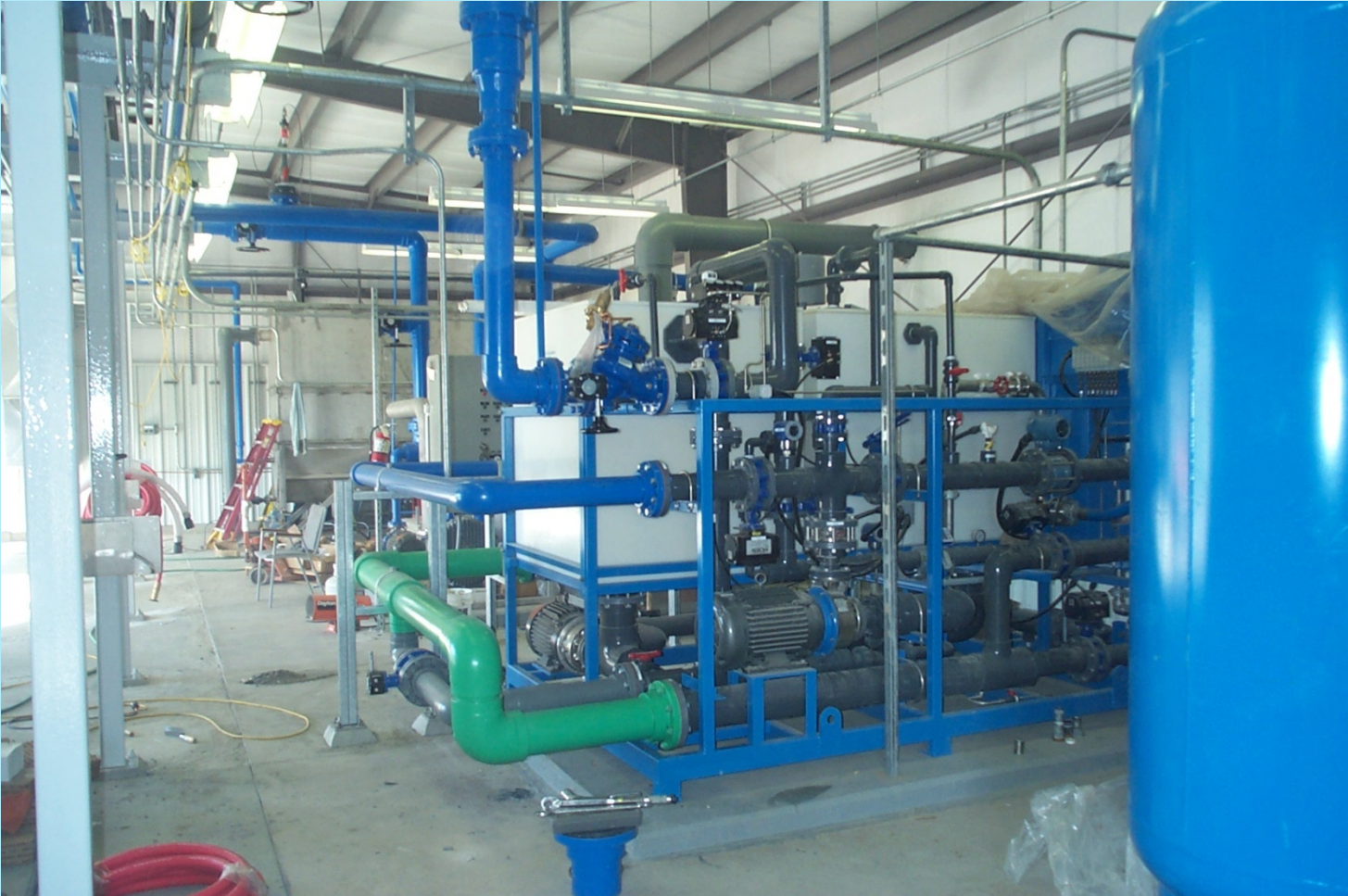
Arsenic Treatment Plant (Fallon Paiute Shoshone Tribe)
